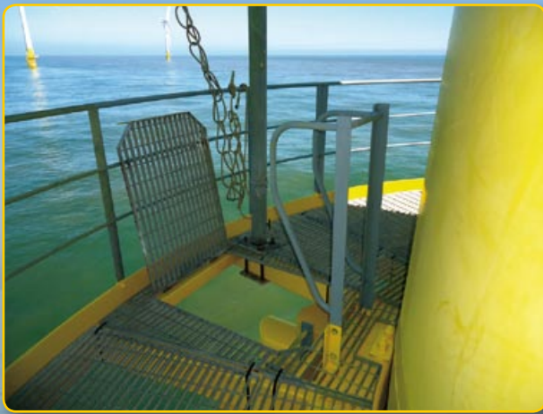
Re-install grating and davit arms.
