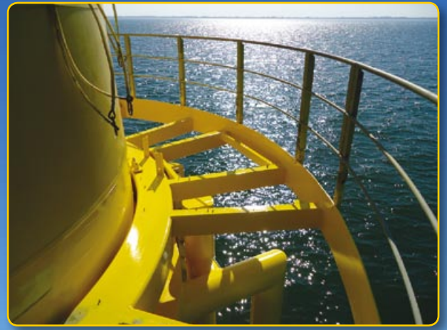
New protective coating applied to top sides of walkway.
