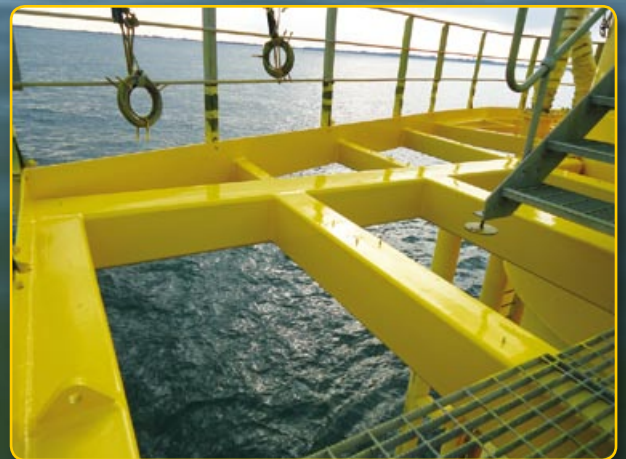
New protective coating, airless sprayed applied to the required thickness.
