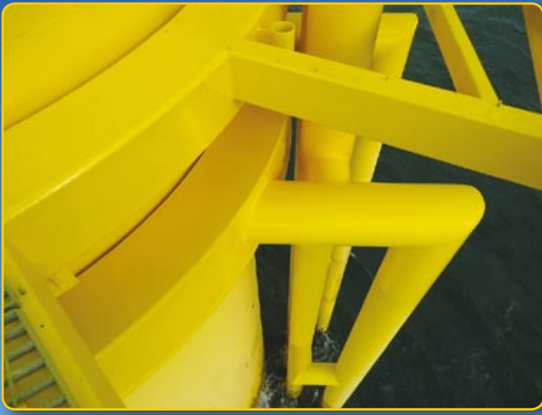
New protective coating applied to underside of walkway.
