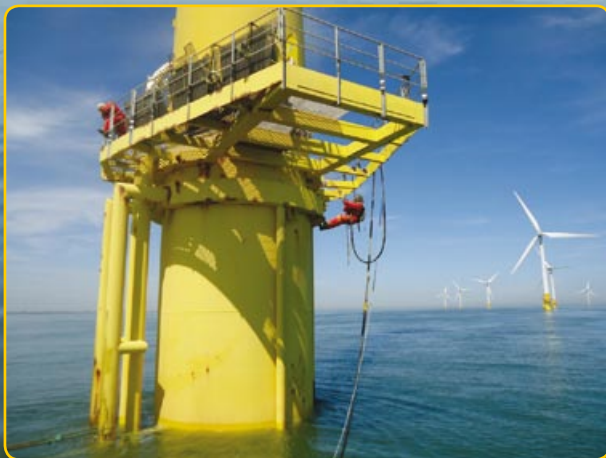
Grit blasting performed using highly skilled roped access techniques
