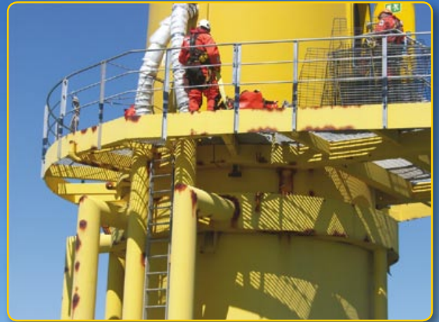
Removal of gratings and davit arms in preparation for grit blasting.
