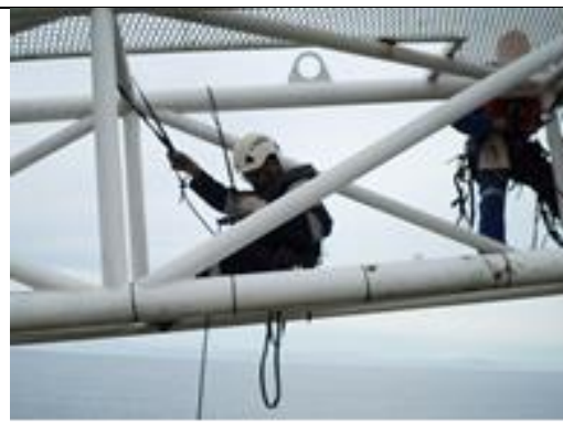
INDUSTRIAL ROPE ACCESS SERVICES
