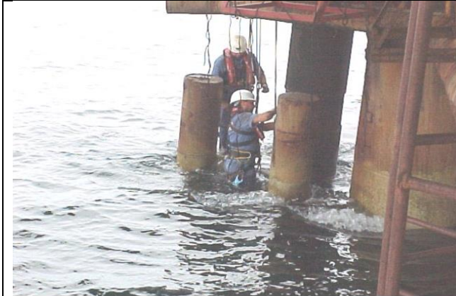
OFFSHORE STRUCTURAL SURVEYS
